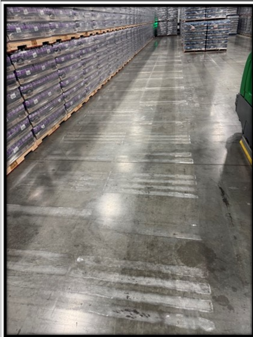
Calcium acetate crystals forming where green wood contacts wet or unsealed concrete floors.
